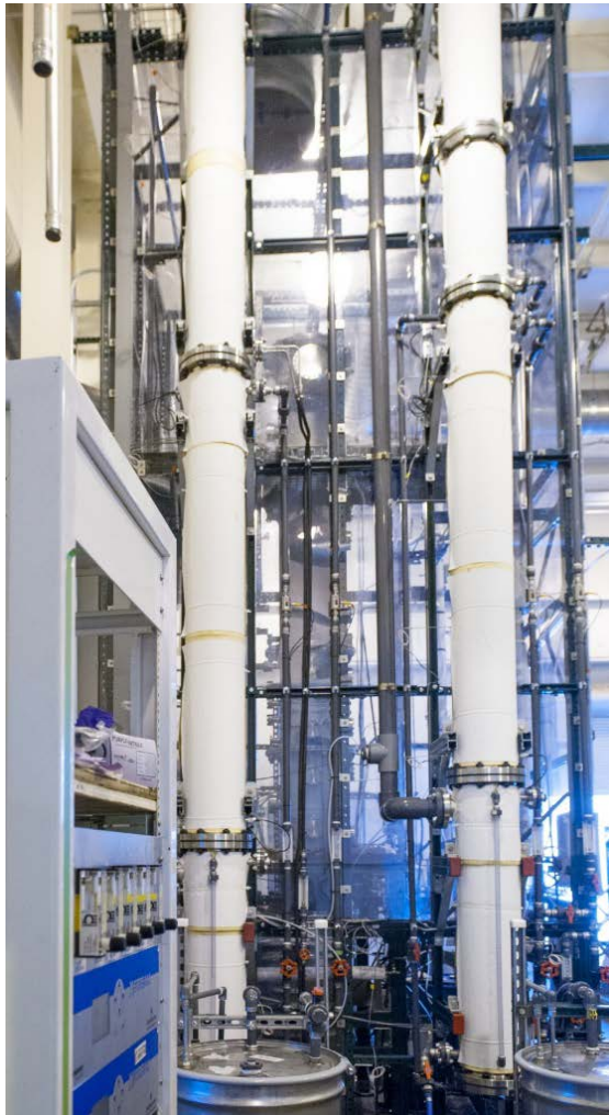
Absorbers (0.25 to 1 t-CO 2 /day capacity)
